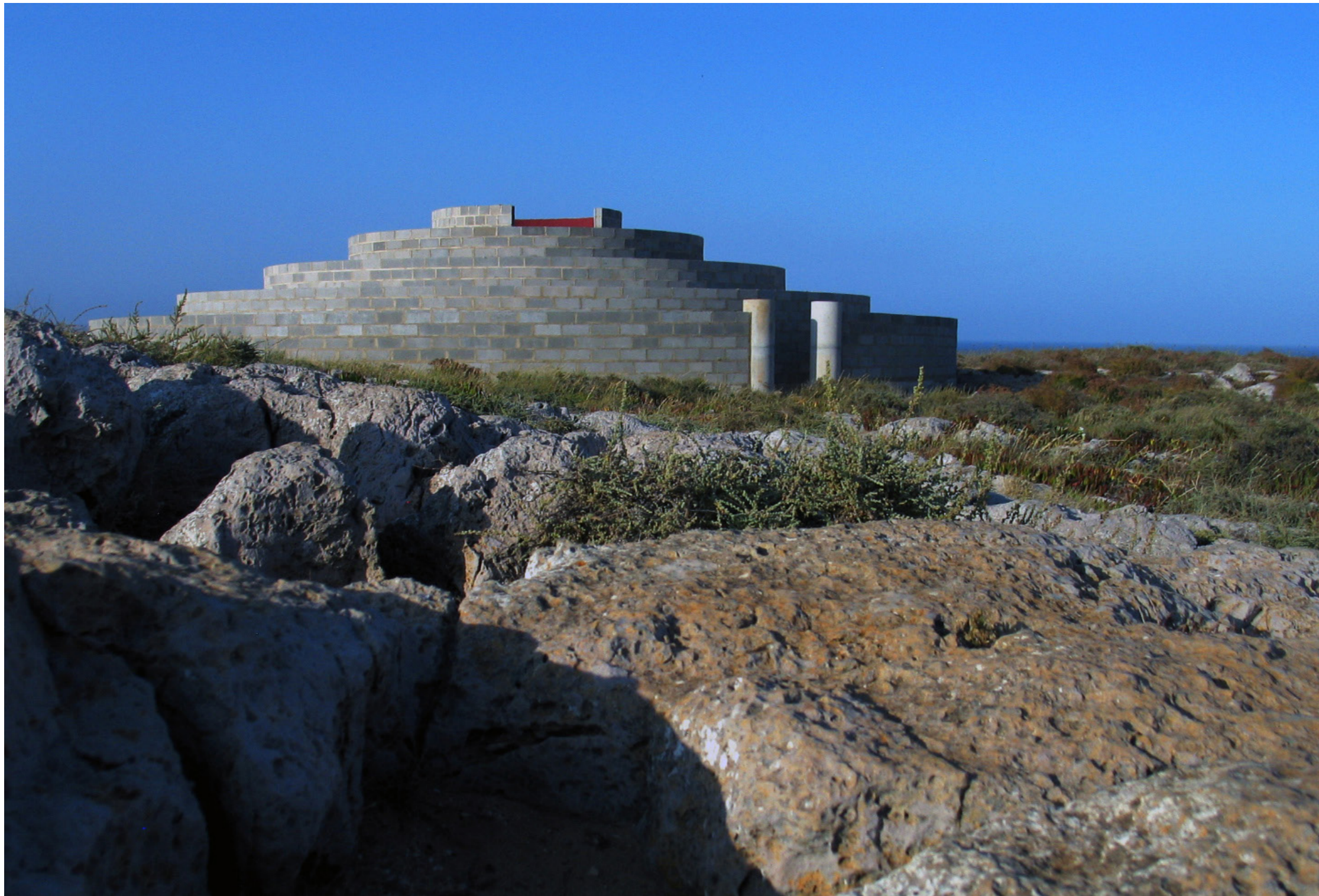
west side - entrance
