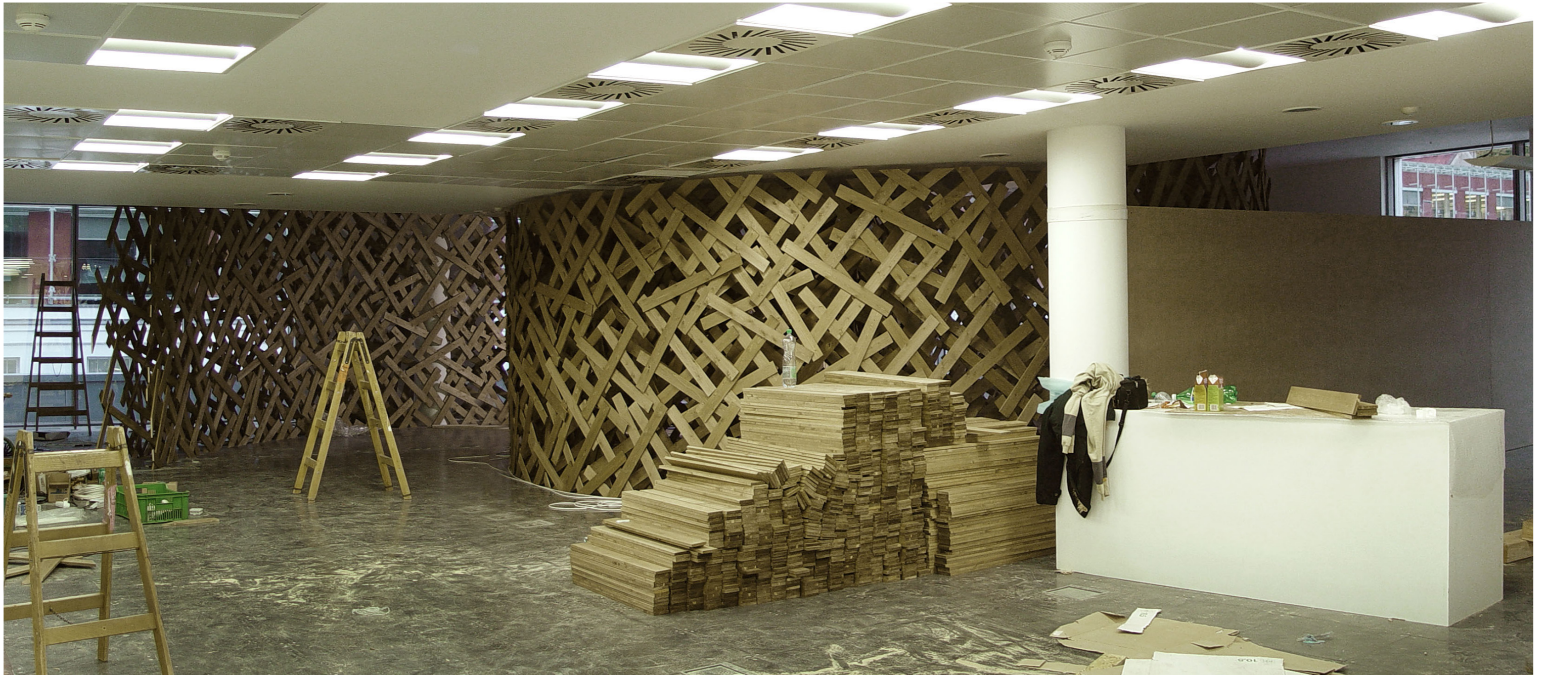
structure was created by wooden slats nailed together
